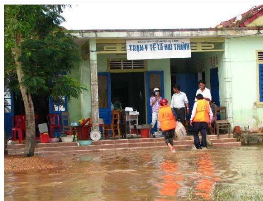
Health care center is submerged
