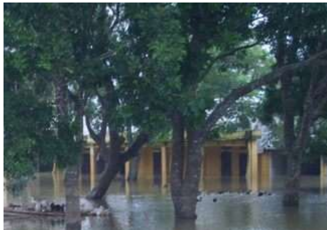
Figure 4: Vinh Khang primary school after 7 day flooded. Ducks are swimming in the play ground
